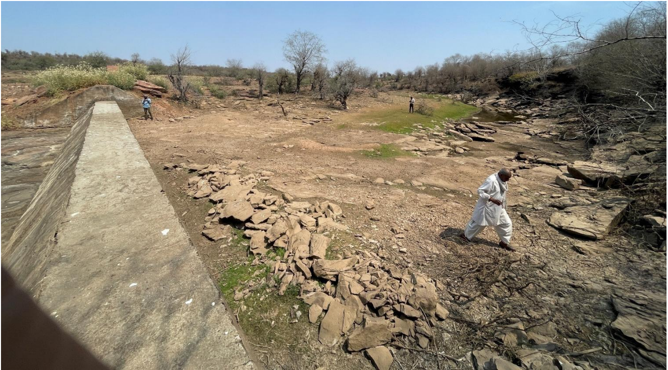
Fig. 6 Core Wall of Karan Sarovar Tal
