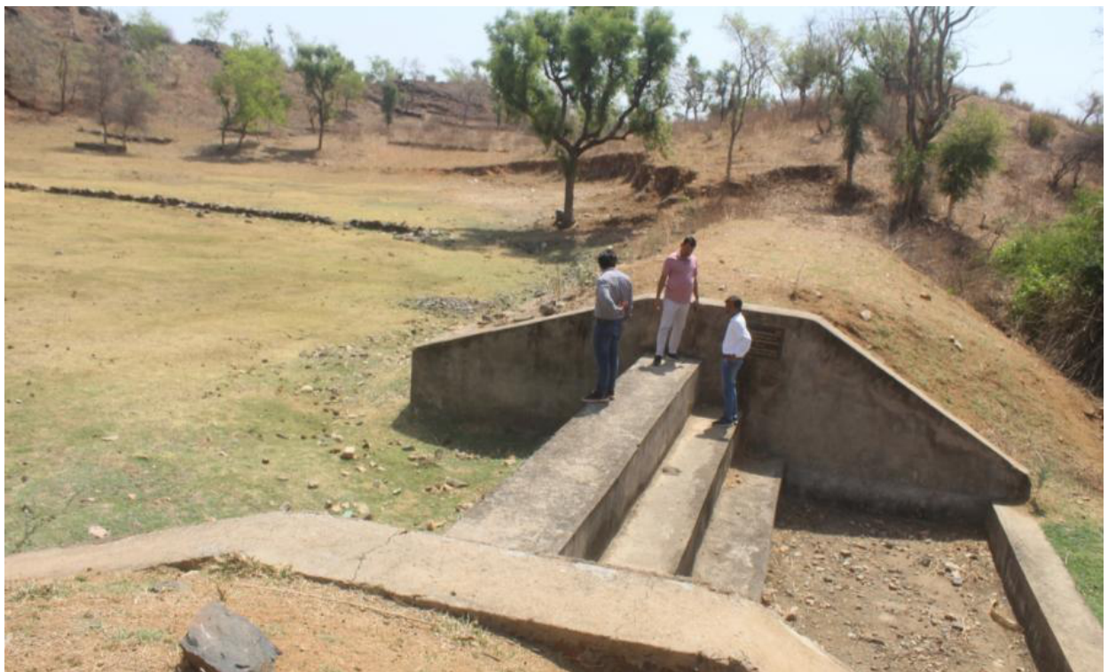
Fig. 60 Earthen embankment with masonry waste weir and stone pitching-2-sagtadi
